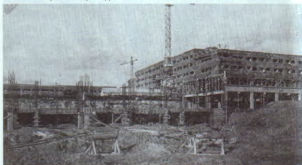
▲ Madrid: City University — Clinical Hospital construction site. Scene of bitter fighting
